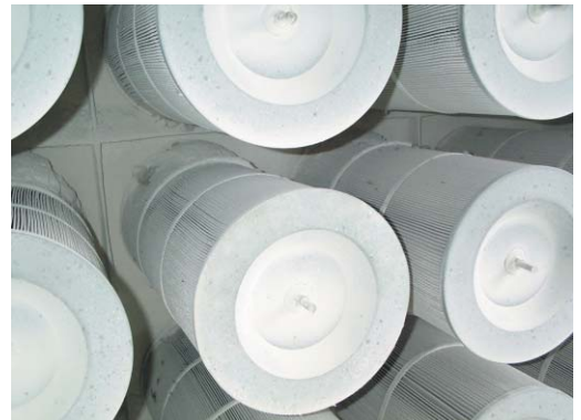
Gas turbine intake air filtration in a chalk plant (GTC 327)
